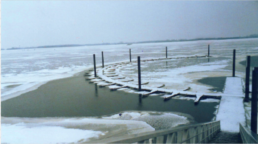
Ice Prevention Plant
