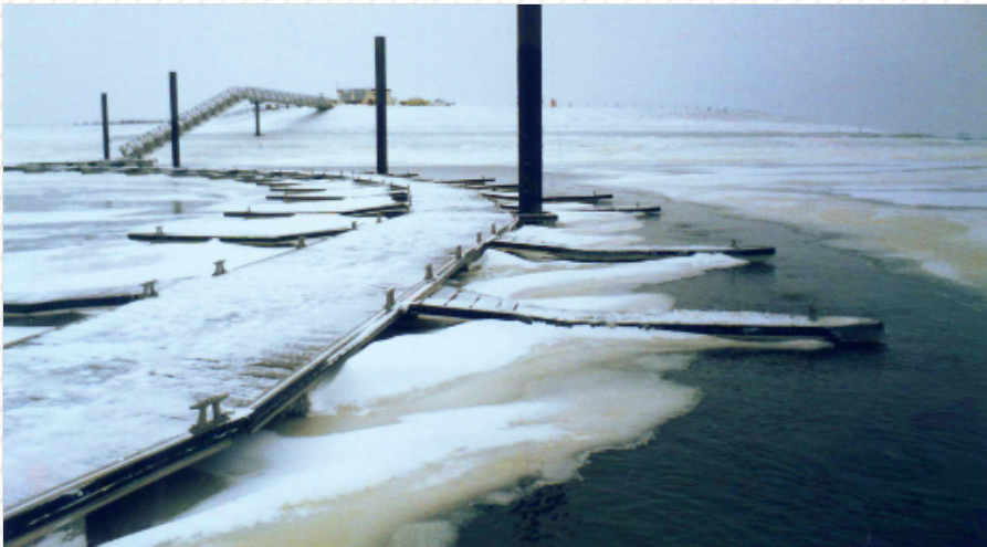
Ice Prevention Plant
