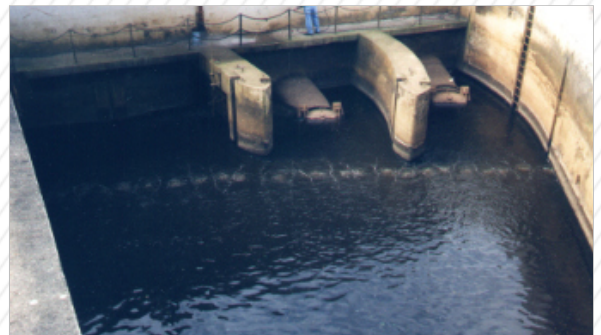
Compressed Air System, Holmer Siel GER
