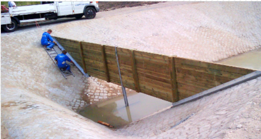
Baffle Board made of oak planks
