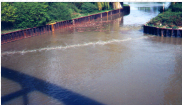
Compressed Air System, Heilbronn GER
