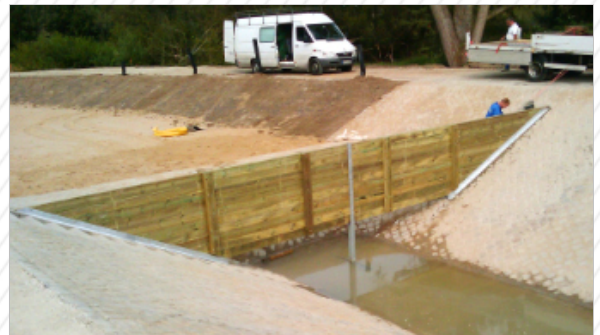
Baffle Board made of oak planks
