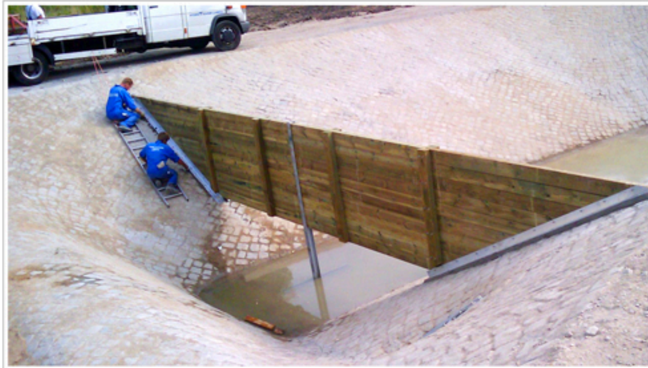
Baffle Board made of oak planks
