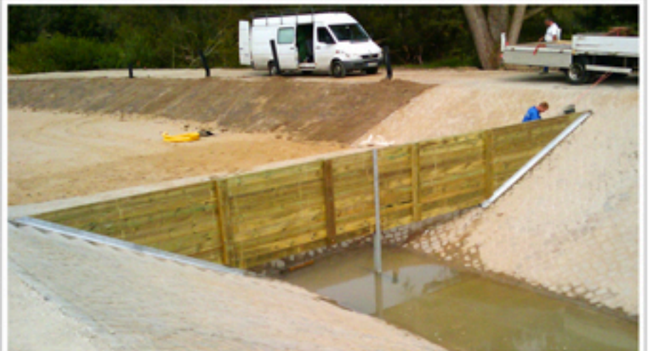
Baffle Board made of oak planks
