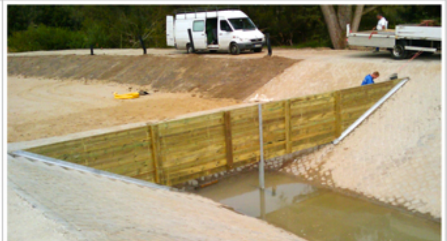
Feste Tauchwand aus Eichenbohlen Baffle Board made of oak planks
